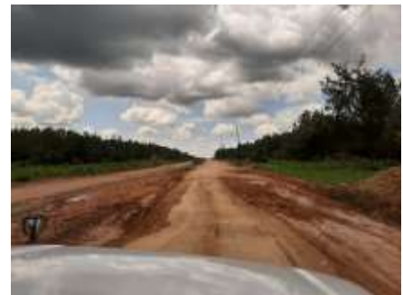
Old road on the left, new on the right... although they don't look much different.
